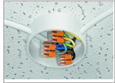
Lighting distribution in ceiling canopy
